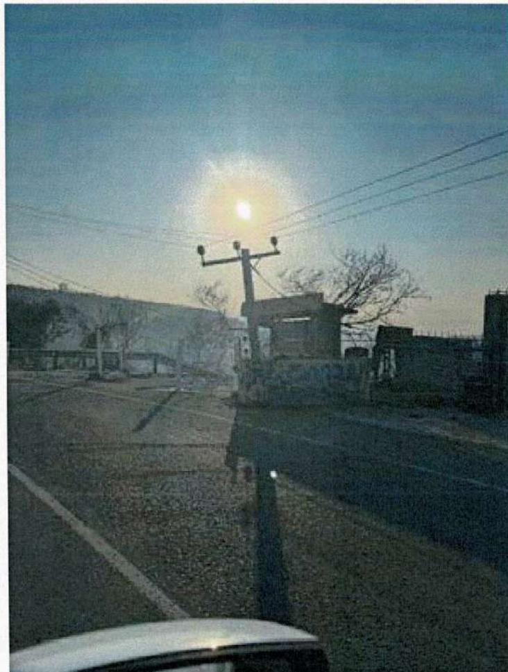
Figure 7: Example of fire damaged electrical infrastructure provided by EAC
